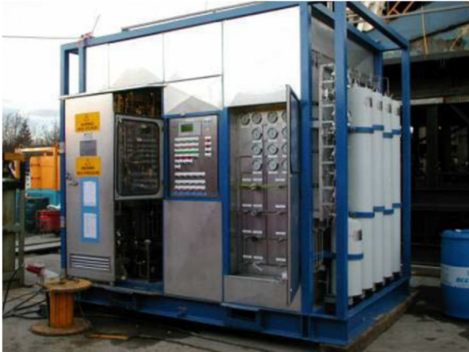
Figure 2.11: Hydraulic Power Unit [Oilfield Wiki].
