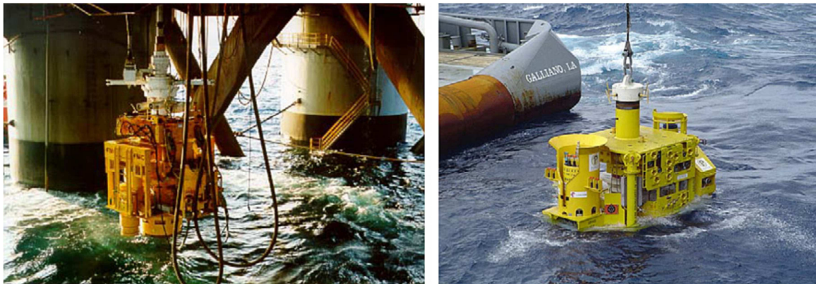
Figure 5-1: Tree Installation by Drill Pipe (Left) and Rig Winch (Right)
