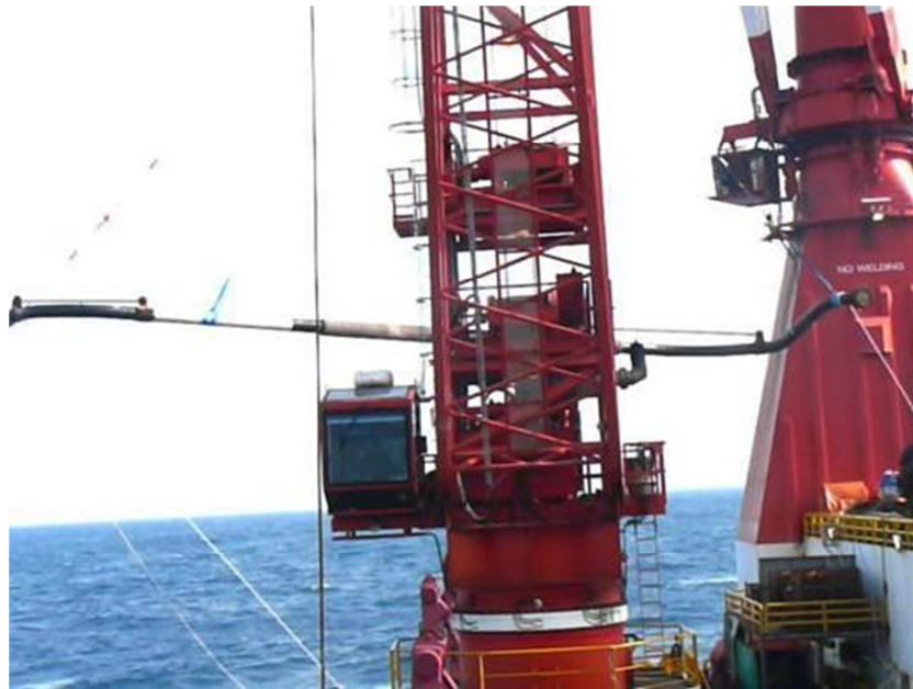
Figure 6.19: Spools installation at site [Zamri]
