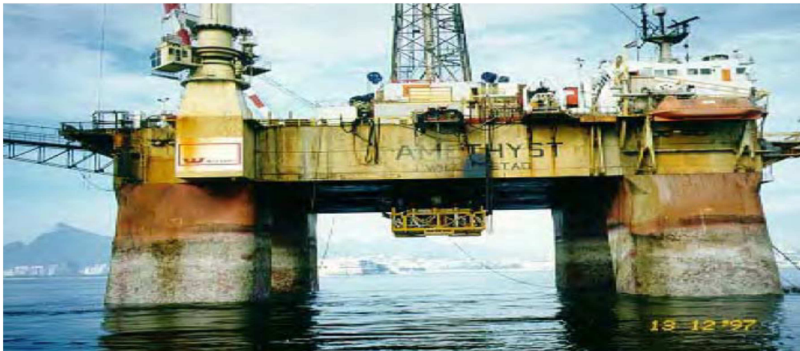
Figure 2.2: Installing Manifold Using Semi-Submersible
