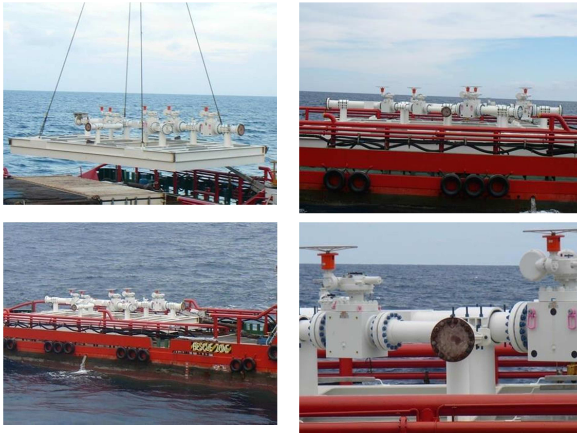
Figure 6.10: Installation of PLEM from barge using crane [Zamri]
