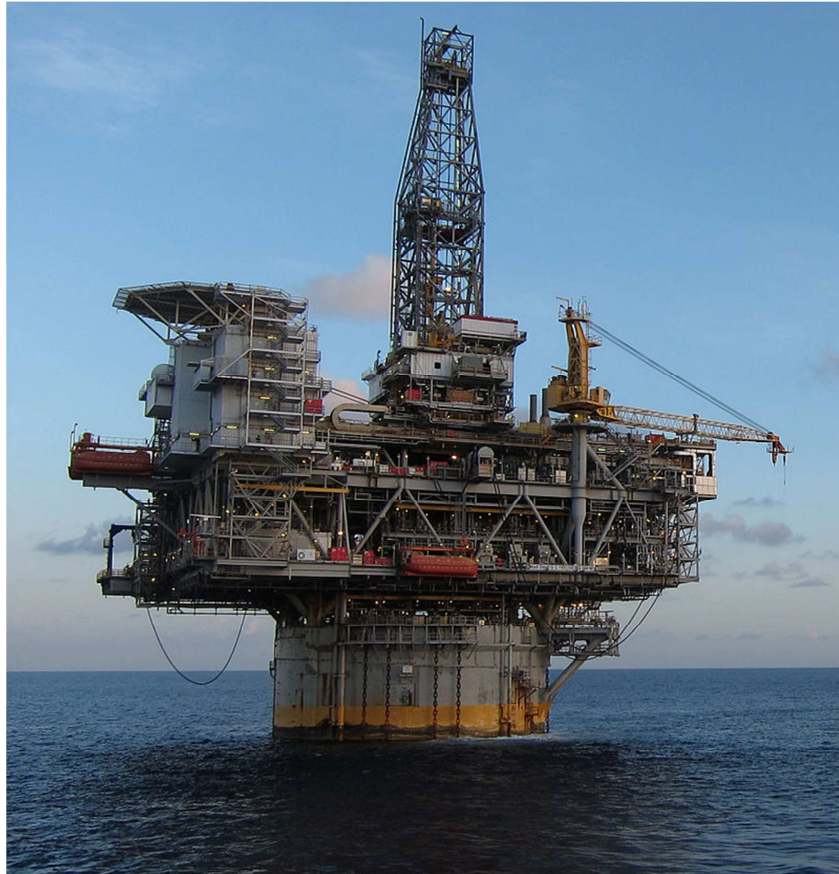
Figure.2.4: Truss SPAR DTU in Kikeh, Malaysia [Koto, 2017].
