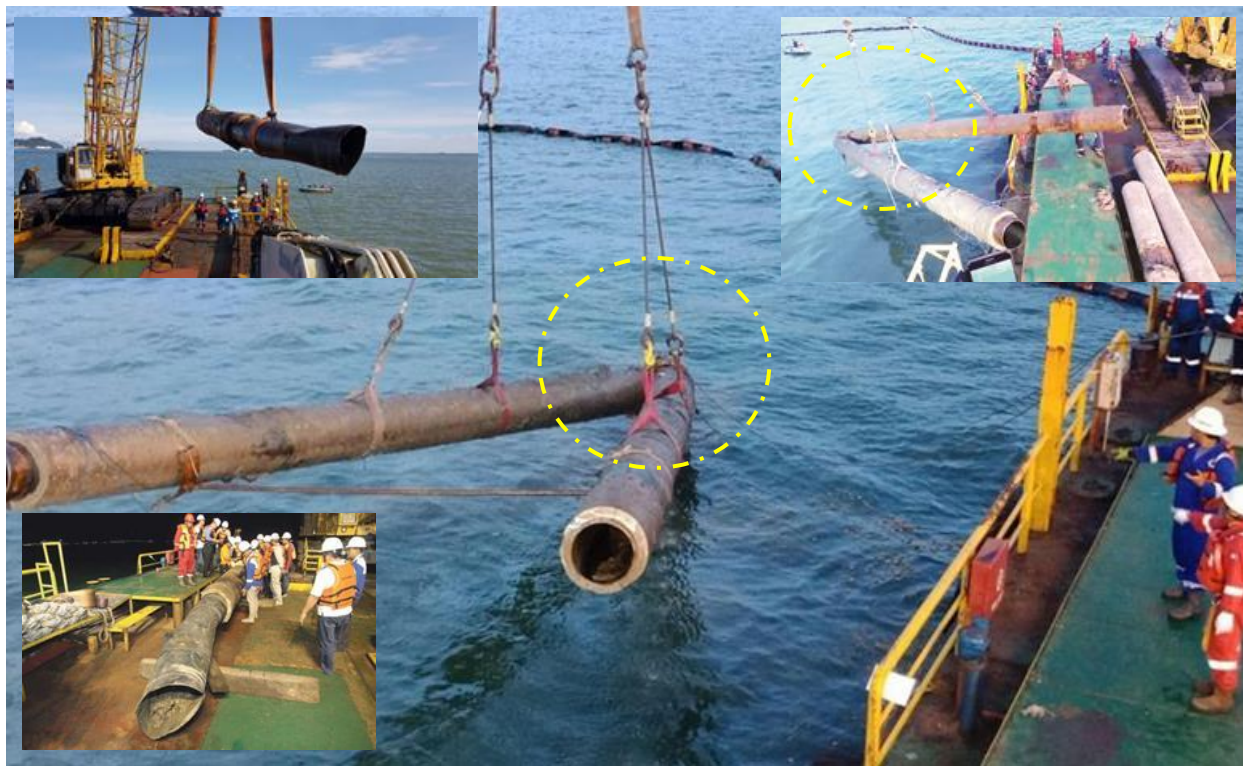
Figure 11: Lifting of subsea pipeline from Sea Heaven.
