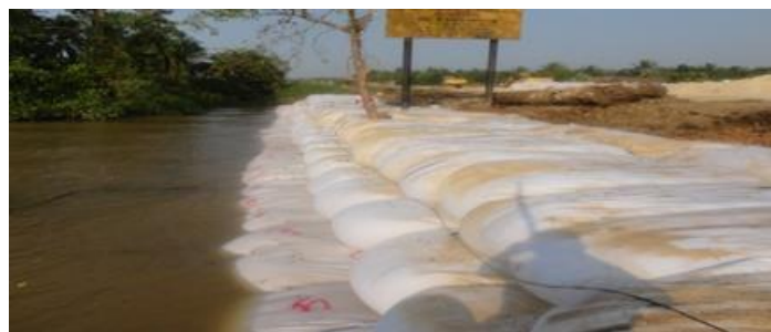
Figure 4: Example of geobag structure in other project site in Indonesia.
