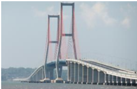
Figure 1: Suramadu Bridge (Source: https://www.pinterest.com )
