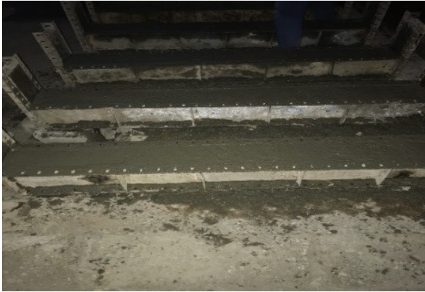
Figure 3: The concrete pouring operations in 8 samples
