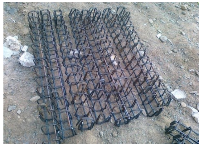
Figure 2: Reinforcement of concrete beams
