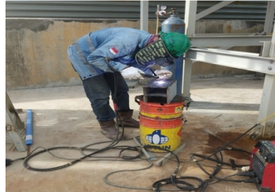
Figure 2: Specimen welding
