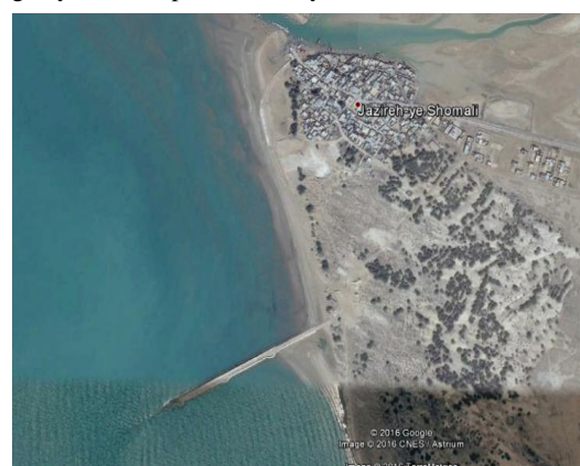
Figure 7: Sedimentation behind the Jazireh-e Shomali-Jonoubi Port's breakwater
