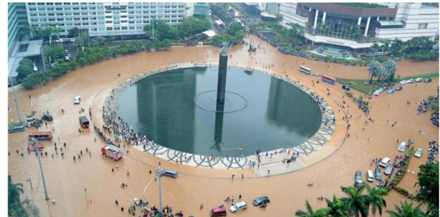
Figure.1.11: Flood in DKI Jakarta 2014 [BNPb].
