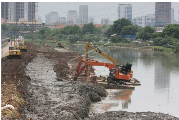
Figure.1.16: Ciliwung River Mud Dredging in DKI Jakarta [DKI Jakarta]
