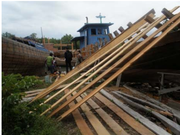
Figure.1: Drying lumber issue in traditional ship production in Kepulauan Riau, Indonesia.
