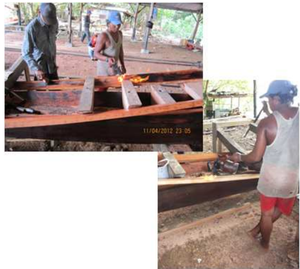
Figure 11: Planks bended using fire technique.
