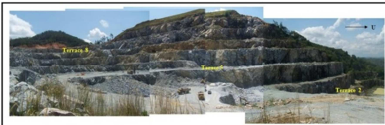
Figure 2: Field study area (terrace) at Kajang Rock Quarry.
