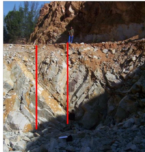
Figure 4: Line of discontinuity in vertical scanning survey.
