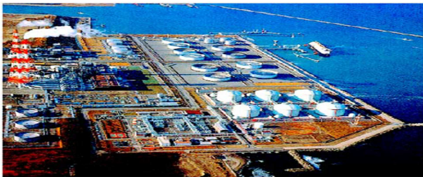
Figure 7: Canaport Receiving / Import Terminal, Canada
