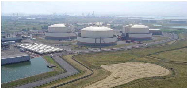
Figure 6: Canaport Liquefaction LNG terminal, Canada (Sheila Goucher, 2013)
