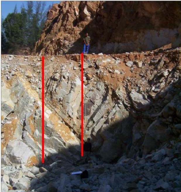
Figure 4: Line of discontinuity in vertical scanning survey.
