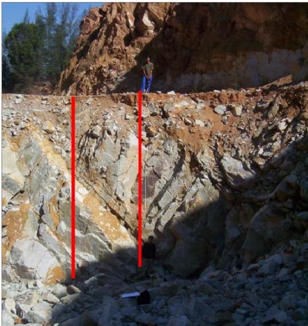
Figure 4: Line of discontinuity in vertical scanning survey.
