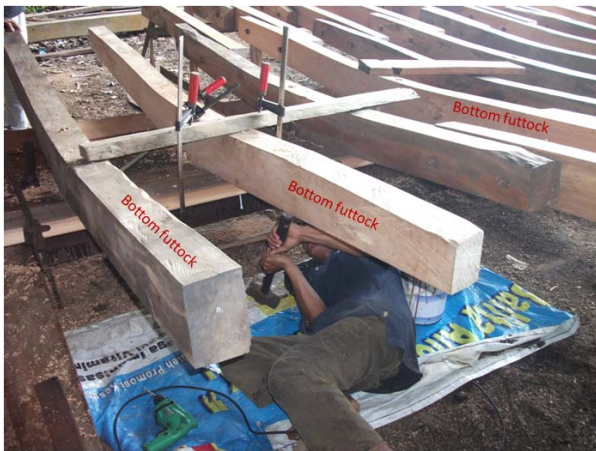
Figure.10: Bottom frames installed on the keel.
