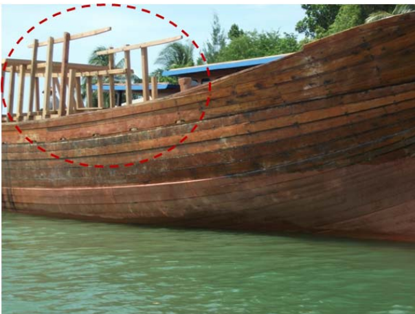
Figure.17: Outfitting and Engine installation.
