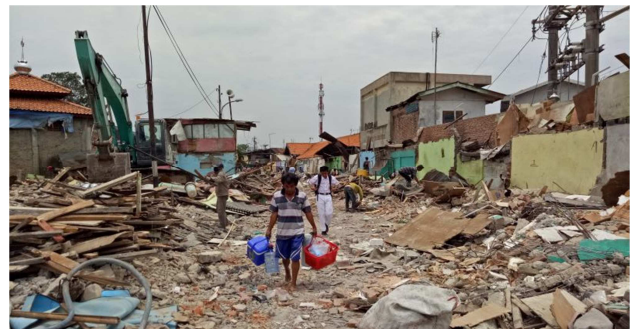
Figure.1.20: he rest of the house from the evictions of residents on Bukit Duri.
