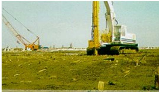
Figure 2: Installation of PVD Fibredrain
